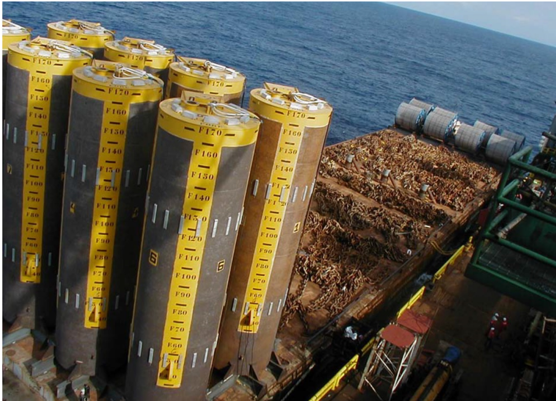
Figure 1.7: Transportation of suction caissons to installation site. Source: Colliat et al. (2011)
