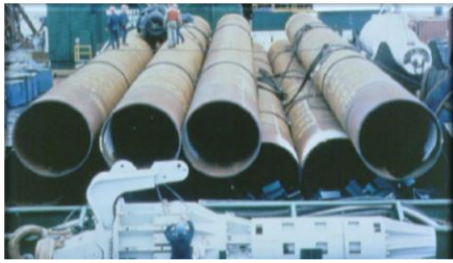
(a) Driven piles (courtesy of JD Murff).
