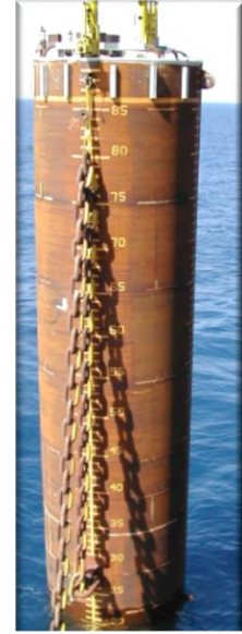
(c) Suction caisson (courtesy of E Clukey).
