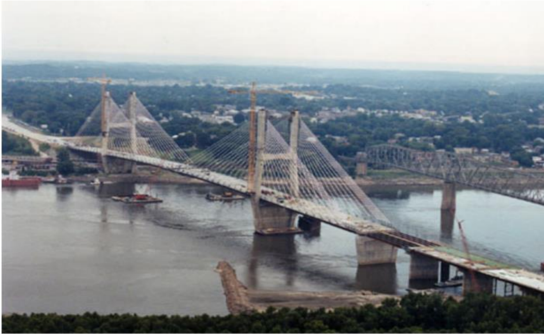
Fig. 4.8: Second Generation Benchmark problem for cable-stayed bridges, located in Cape Girardeau, MO. Reprinted from Caicedo and Dyke (2004).
