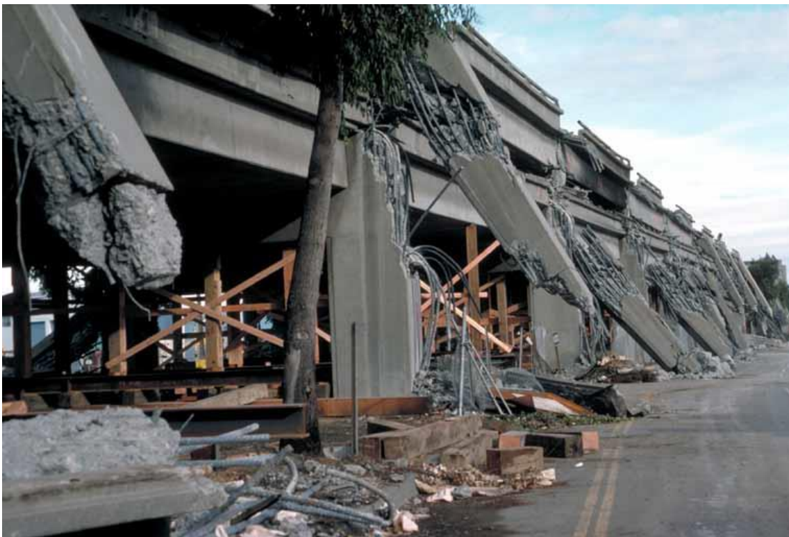
Fig. 1.1: Street Viaduct, Oakland-CA after Loma Prieta Earthquake, reprinted from United States Geological Survey (1999).
