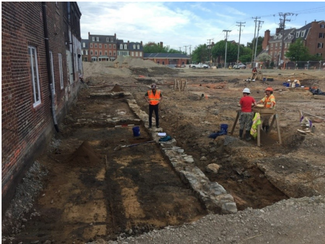
Figure 12. Hooe's Warehouse and Store. Remains of warehouse stone foundation. Photo courtesy of Alexandria Archaeology.
