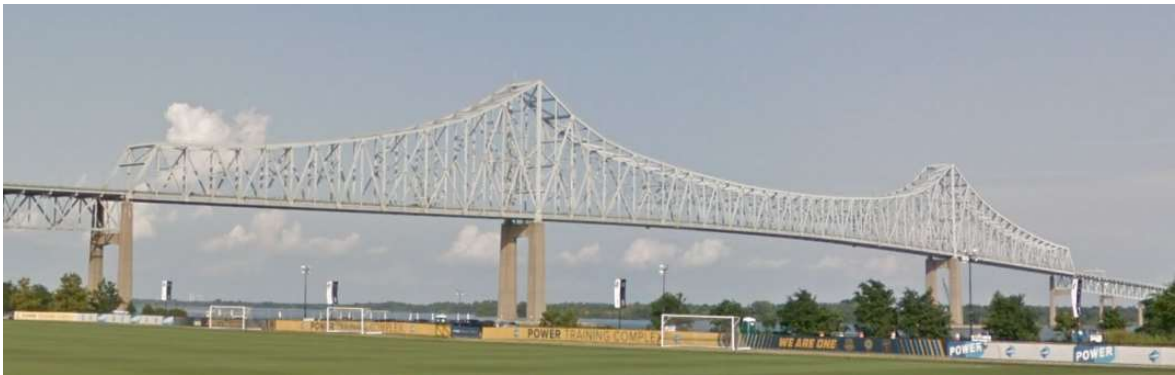
Figure 116: Commodore Barry Bridge (Courtesy of Google Maps)
