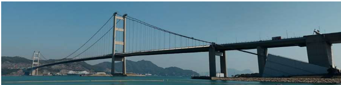
Figure 121: Tsing Ma Bridge (Courtesy of Google Maps)
