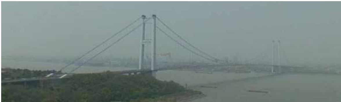
Figure 119: Jiangyin Yangtze River Bridge (Courtesy of Google Maps)
