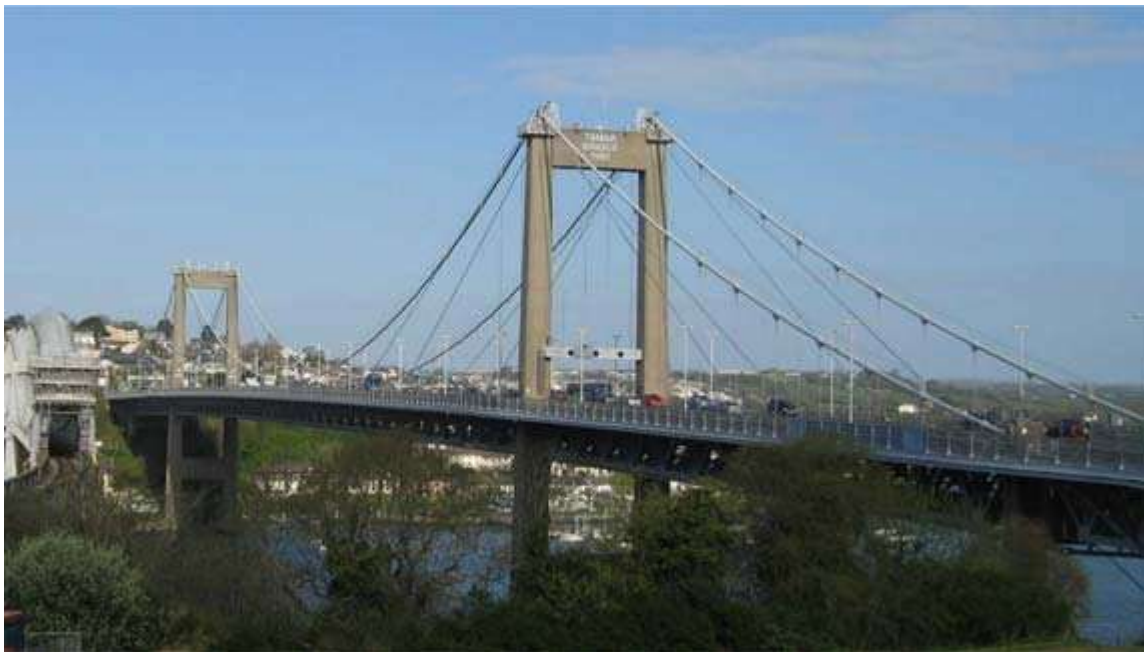
Figure 122: Tamar Bridge (Reprinted from Jesus et al. 2018)
