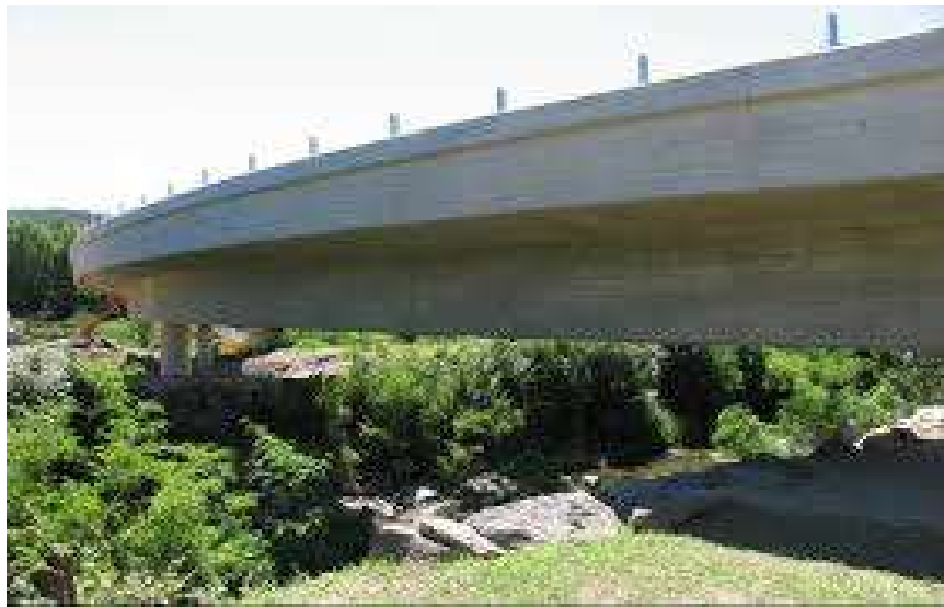
Figure 112: Ricciolo Vedeggio Viaduct (Reprinted from Glisic et al. 2008)
