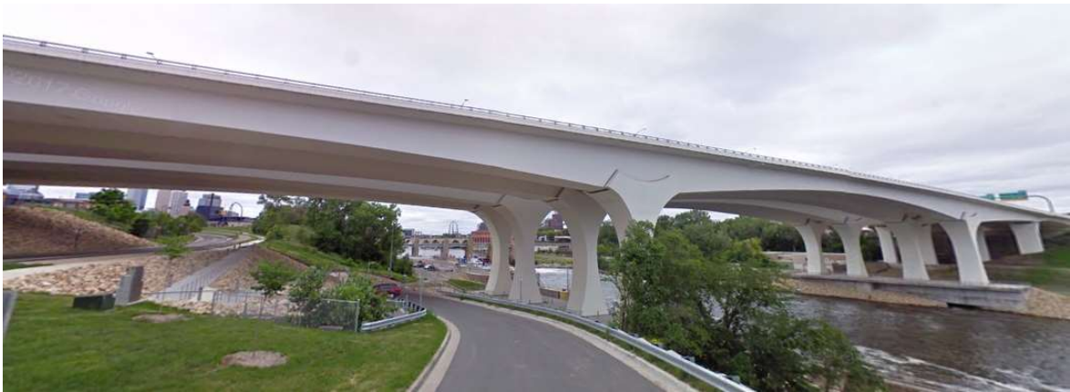
Figure 115: I-35W St. Anthony Falls Bridge (Courtesy of Google Maps)
