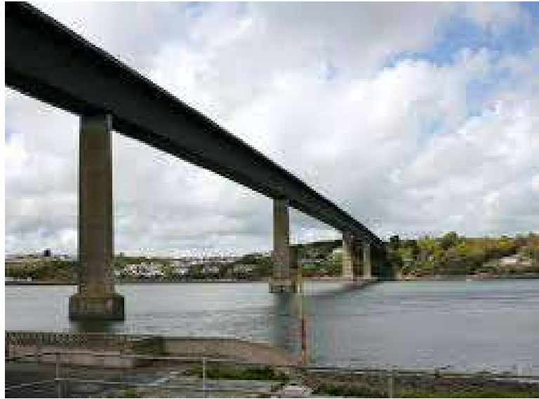
Figure 117: Cleddau Bridge (Reprinted from Kromanis and Kripakaran 2014)
