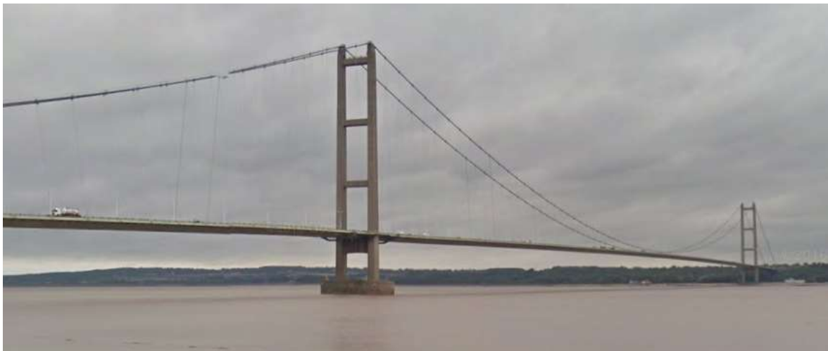
Figure 123: Humber Bridge (Courtesy of Google Maps)
