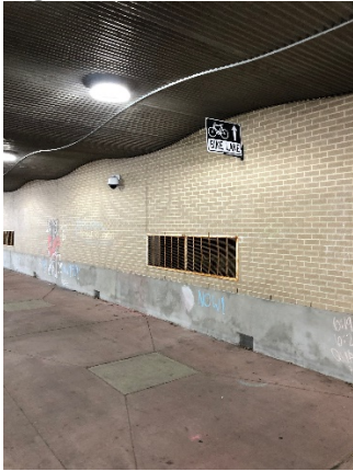
Figure 4.8. Photo with Less Visible Bike Lane Signage on Route 1.
