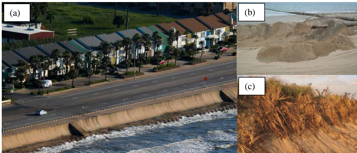
Figure 1.1: Three methods to reduce the risk for flooding and flood-related damages along coastlines. The Galveston Seawall is shown in (a) (Snyder, 2017). (b) shows sand being pumped from offshore onto an eroded beach for a beach nourishment project, image courtesy of SCEhardt. (c) displays a vegetated sand dune (Feagin et al., 2015)
