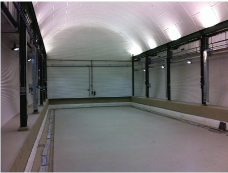
FIGURE 19: View of Hall A of the Laboratorio Subterráneo de Canfranc prior to any equipment installation.
