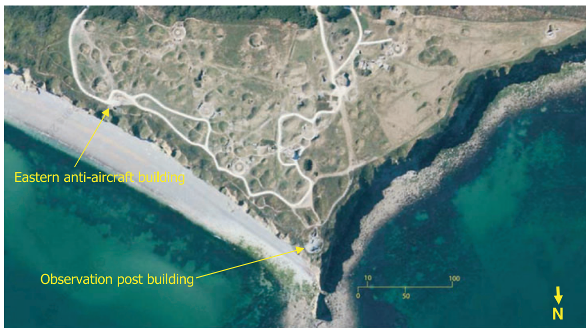
Figure 2. An aerial view of Pointe du Hoc showing locations of the two major at-risk buildings.
