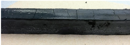
FIGURE 5: A beam made from batch 9, 24 hrs after casting and immediately after demolding. Batch 9 beams were produced in the same condition (no curing) and with the same mix proportions as those of the beams shown in Figure 4 ( w/c = 0.40 , with silica fume to cement ratio of 20 wt%). The only difference is that batch 9 contains CNF with the concentration of 1.0% of cement mass. There are only very shallow shrinkage cracks at the surface. The beams did not break through any of those cracks during bending test.
