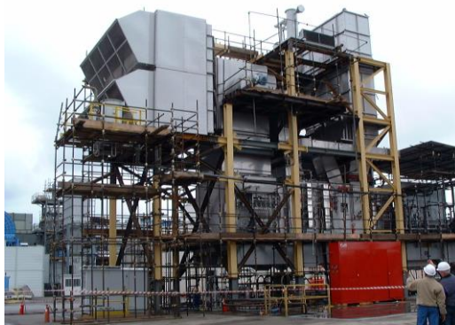
Figure 28: Gas Turbine Offshore Modular Arrangement
