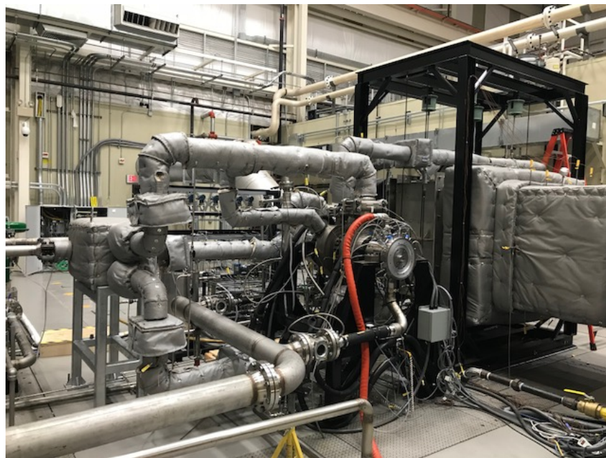
Figure 17: SunShot Turbine Assembly with Insulation
