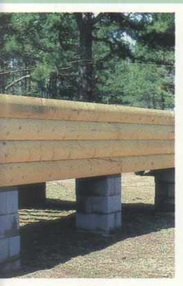
Clearance between the ground
