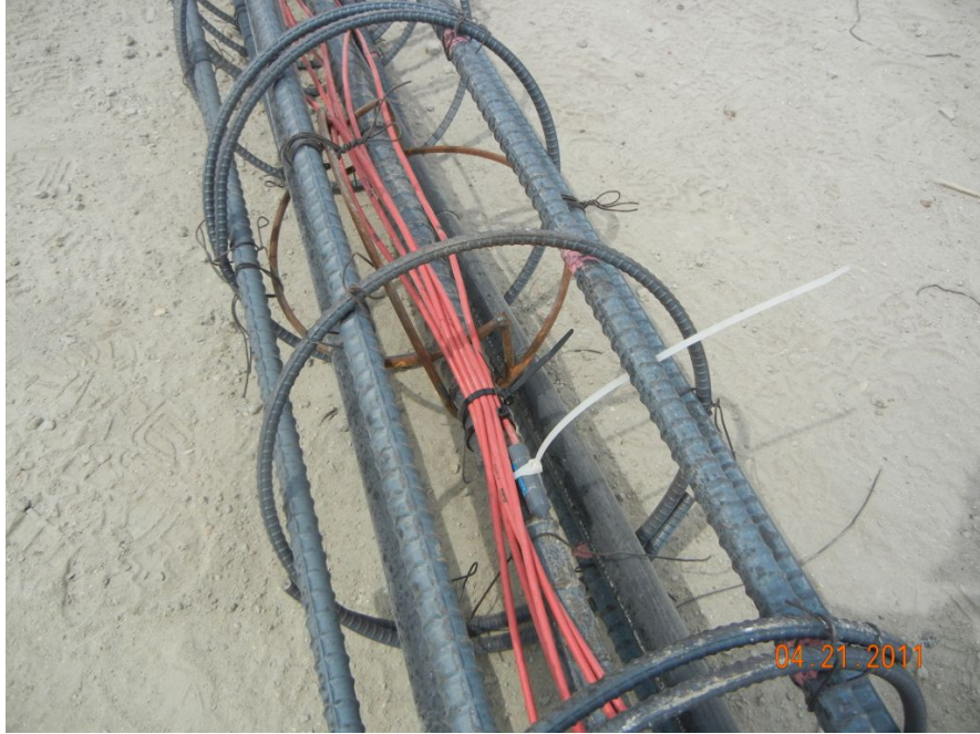
Figure 2.1. Geothermal loops inside the cage of an auger cast pile (Akrouch, 2013)
