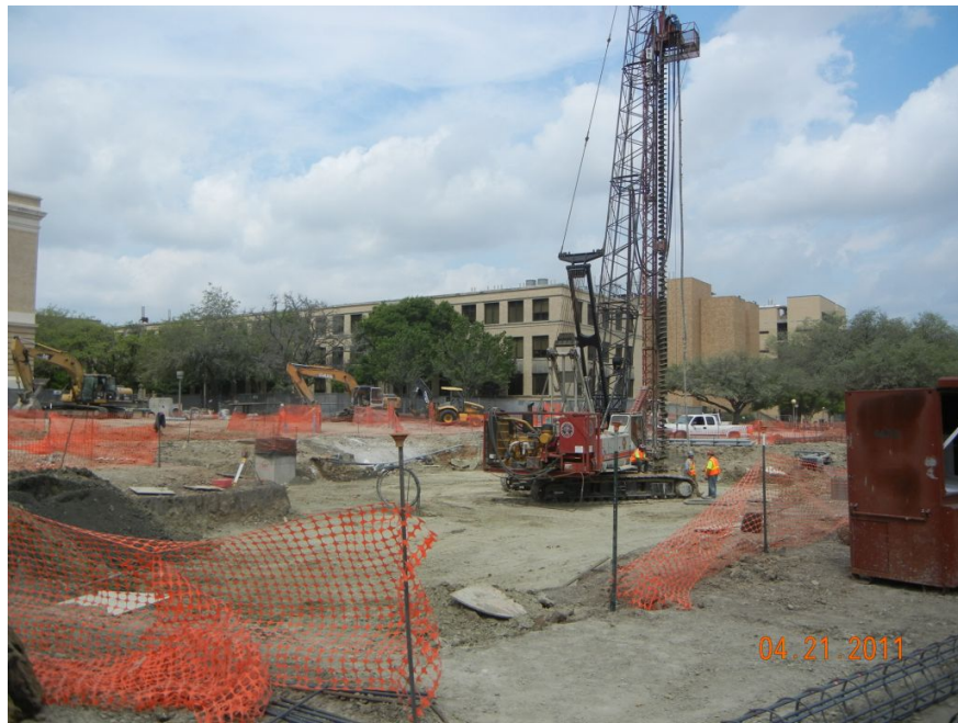
Figure 2.2. Geothermal piles installation (Akrouch, 2013)
