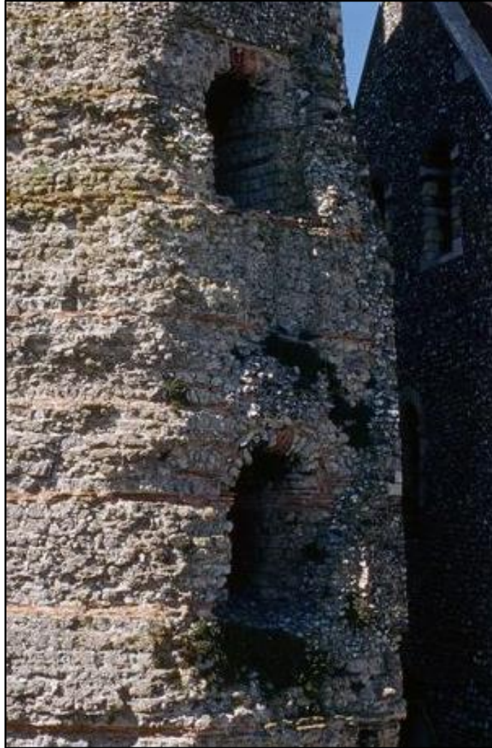
Fig. 2-7. Alternating stone and brick in the arch of a window in the Dover lighthouse. Reprinted with permission from the Hartill Archive of Architecture and Allied Arts, https://library.artstor.org/asset/HARTILL_12312439 (Accessed 10/23/2018).
