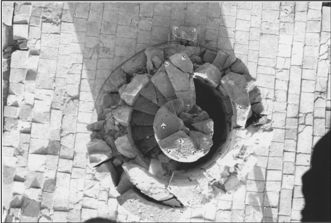
Fig. 3-8. Inner and outer cylinders and staircase of the Patara lighthouse. Reprinted from İşkan-Işık et. al. 2008, 120.
