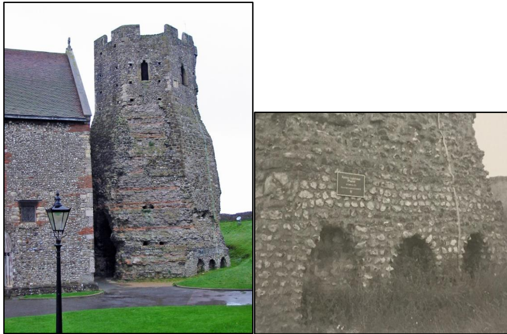
Fig. 2-8. Possible pilae of the Dover lighthouse. Left: reprinted under a Creative Commons license ( https://creativecommons.org/licenses/by-sa/4.0 ), photograph by Chris McKenna (Thryduulf), 2004.
