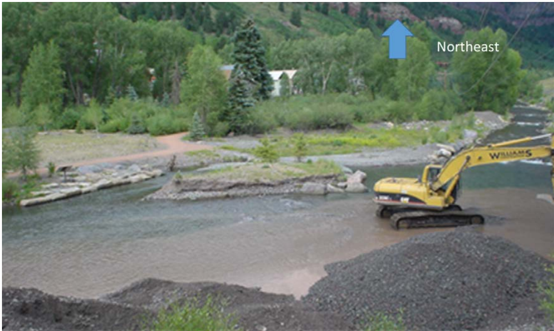
Figure 23: Excavation and maintenance of Instream Sedimentation Basin, 2003.
