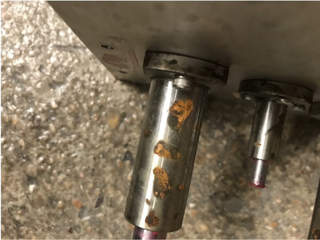
Figure 3.12: Oxidation on the outside of the linear bearings
