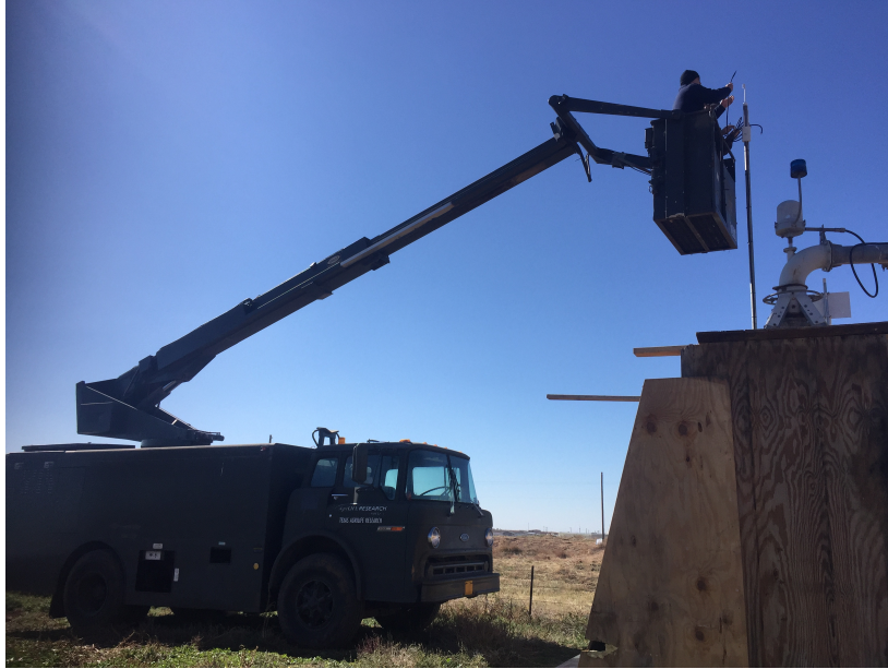
Figure 5.6: An antenna was mounted at pivot, high enough to have clear line of sight to GPS and sensors.
