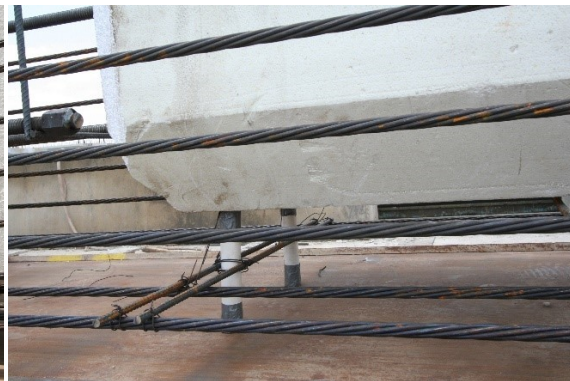
(b) PSV-28B PVC Drain Pipes
