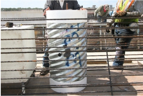
(a) PSV-28A Corrugated Pipe Secured to Prestressing Bed
