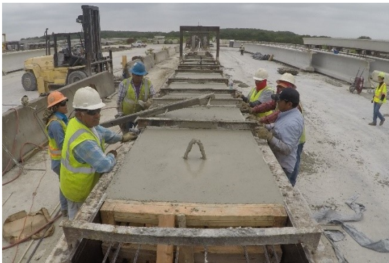
(c) Removing All-Thread Rods Securing Polystyrene Voids
