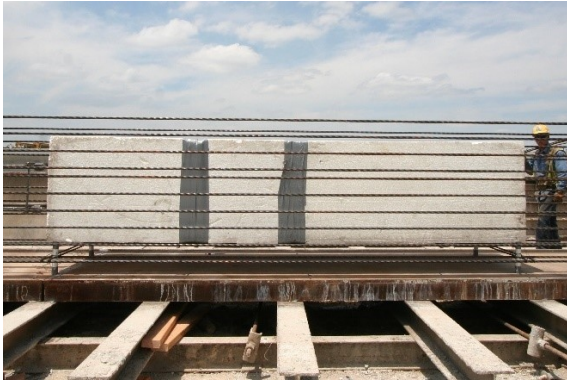
(a) PSV-28A Interior Void Polystyrene Block – In Place
