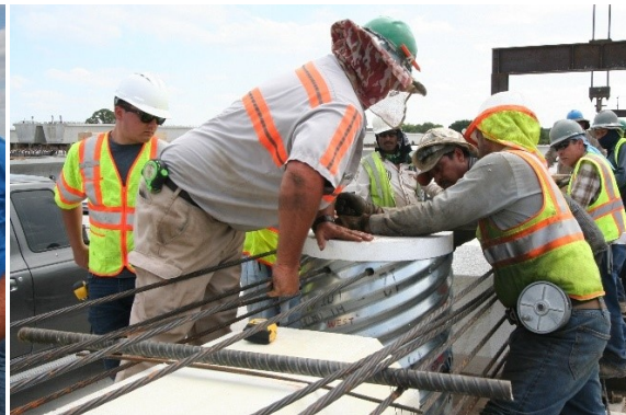
(b) Workers Feeding Strands Through PSV-28B Pipe
