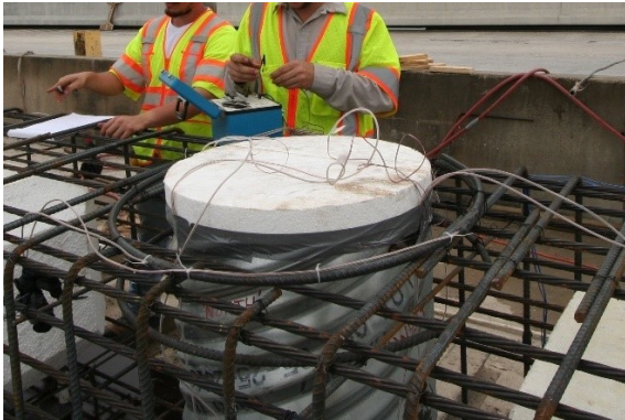
(b) Hoops at Top of Steel Pipe
