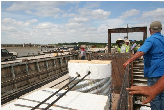
(a) Strands Placed Through PSV-28A Forming Plug
