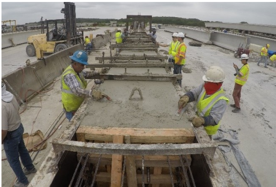
(a) Trowel Finishing
