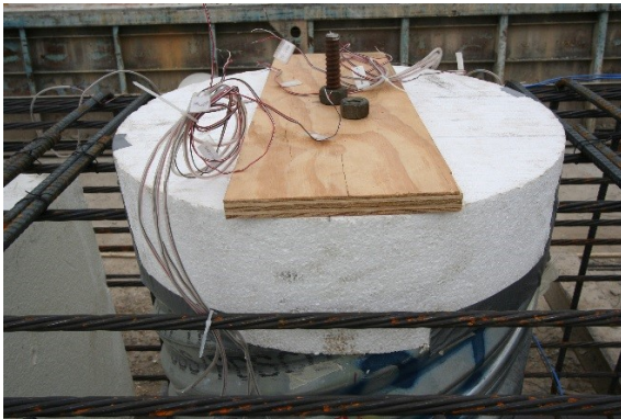
(c) PSV-28A Polystyrene Plug Secured with All-Thread Rod
