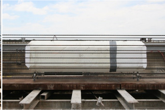
(b) PSV-28B Interior Void Polystyrene Block – In Place
