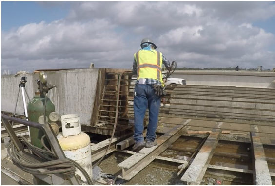
(a) Torch Cutting Strands
