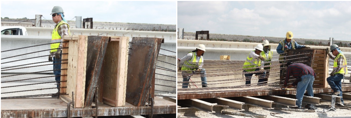
(a) Prior to spreading headers
