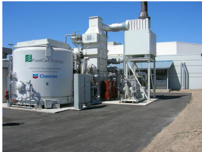
b) Fuel cell as part of Santa Rita Jail microgrid
