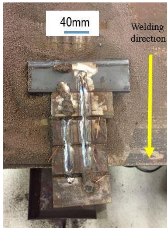
Figure. 4.2. Welding speed calibration.
