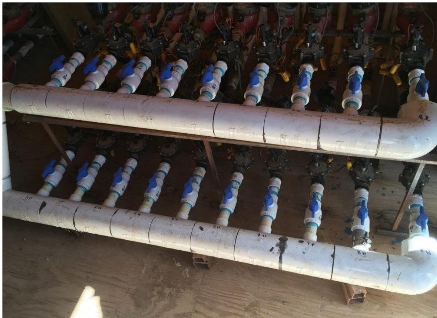
Figure 3. Valve Hub Used to Deliver Specified Irrigation Amounts to Drip Feeds in Experimental Field.
