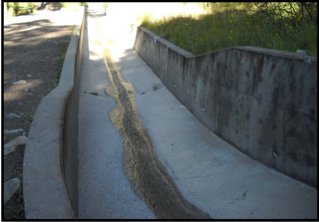
Figure C-3: Cascade creek flume built to divert and minimize hazards from debris flows.
