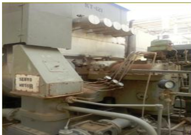
Figure 10. Old Mechanical Governor and Hydraulic Actuator.
