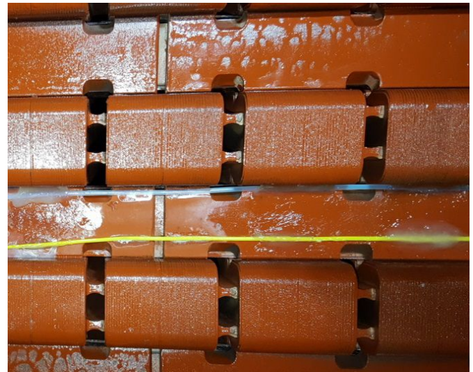
Fig. 19 - Top view of the core slot where the two Brillouin sensing arms are laid onto the wedge.
