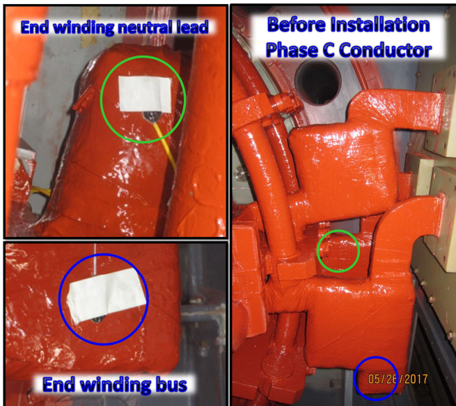
Fig. 10 – Two discrete sensors coupled at two different locations of the neutral bus of the phase C conductor.
