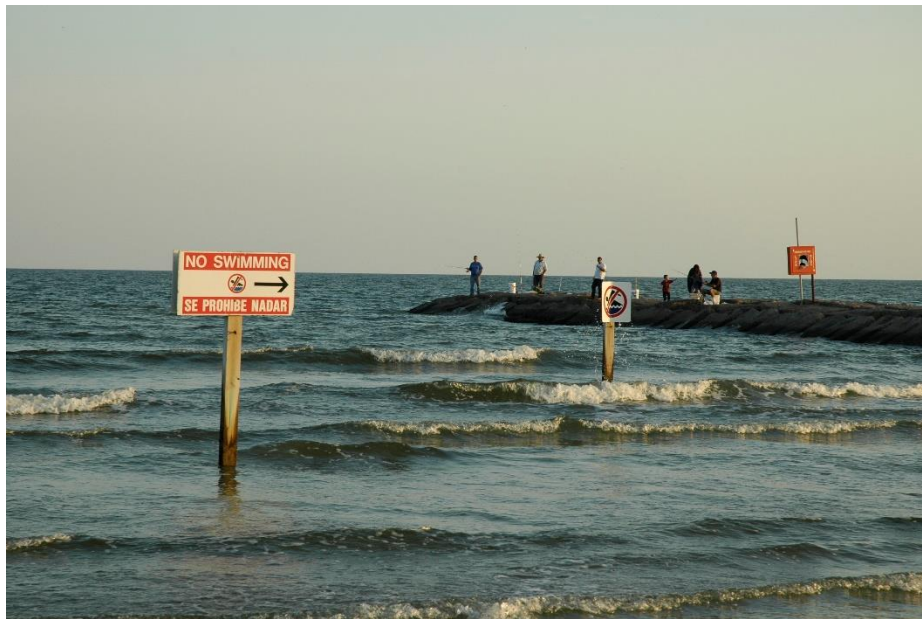
Figure 9 Picture of a “no swimming” zone enforced adjacent to groins at Galveston Beach, Texas, USA because of the rip current that is often forced against the groin when large enough waves are present.
