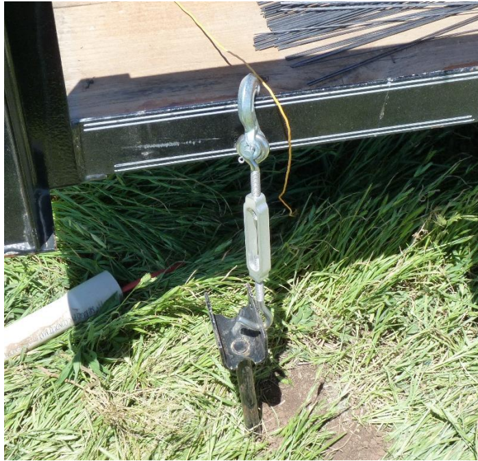
Figure 13. Turnbuckle and anchor system used to secure the trailer in place.
