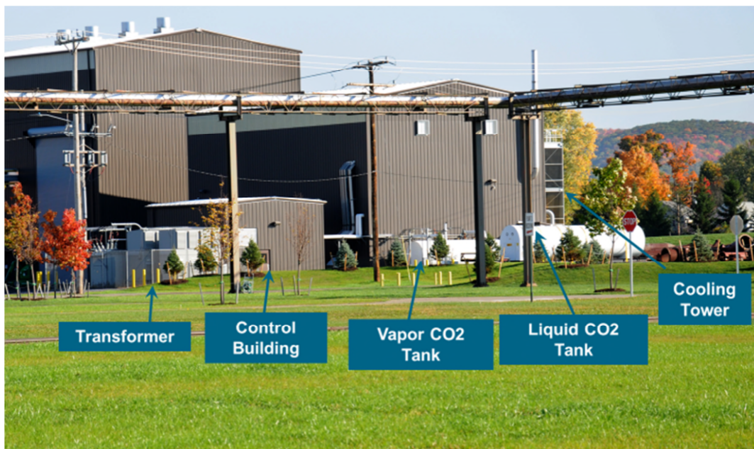
Figure 10. High-pressure CO 2 compressor test facility.
