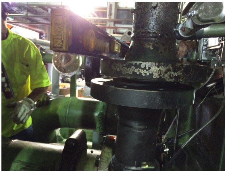
Figure 9: Piping Misalignment
