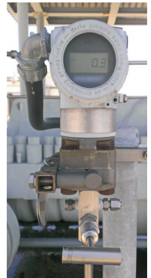
Figure 3 Transmitter with local indicator
