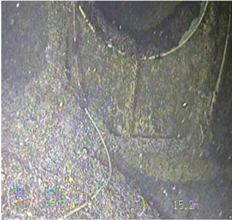
Significant marine fouling
