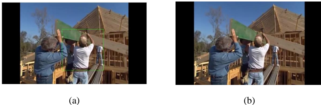
Figure 45 Example of a false negative. (a) True positive made by PARS; (b) false negative made by PTARS because it failed to detect the hammer within the potential tool area.
