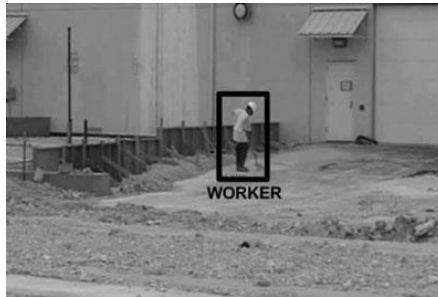
Figure 5 Illustration of a worker detection result. A worker was detected and circled in an image captured by a standard video camera on a construction jobsite (reprinted from Chi & Caldas, 2011).
