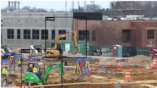
Figure 8 Detection of multiple excavators and construction workers (reprinted from Memarzadeh et al., 2013).
