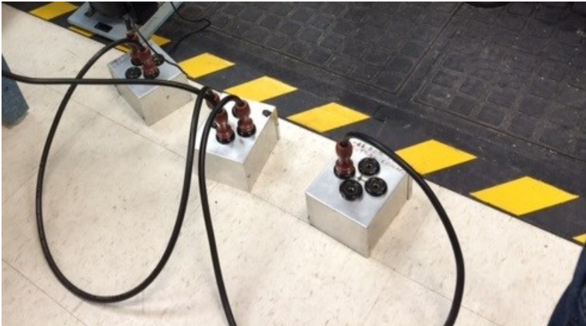
Fig 2.18: Ground connections of the system.
