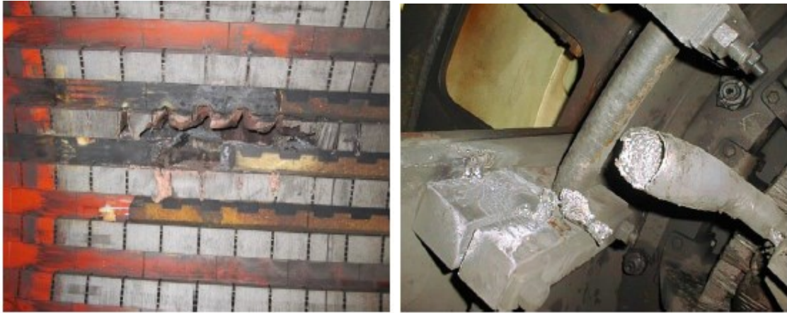
Fig. 1.1: Stator windings insulation failure.
