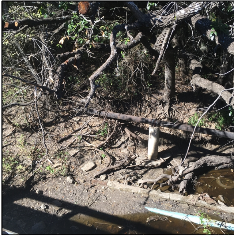
Figure 8. Aerial pipe and partially buried water line
