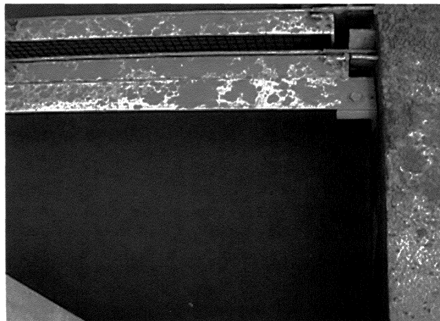
Figure 19. View of Suction Inlet Area.
