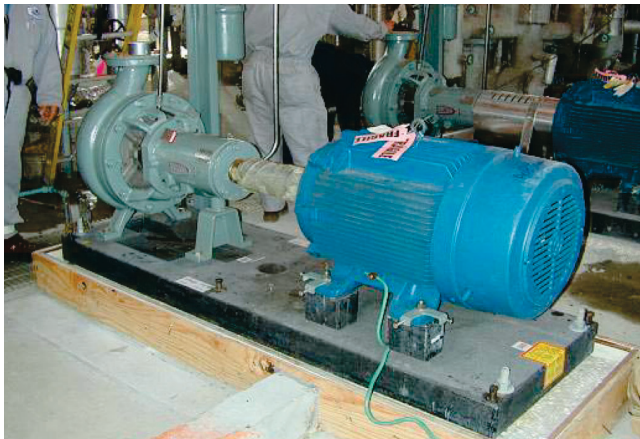
Figure 5. Polymer Concrete Baseplate During Installation.
