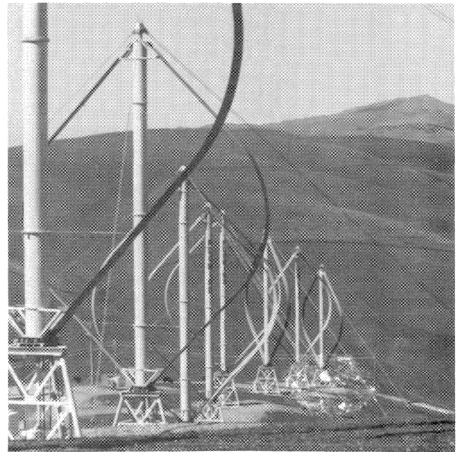
Figure 5. Typical Vertical Axis Machine.
