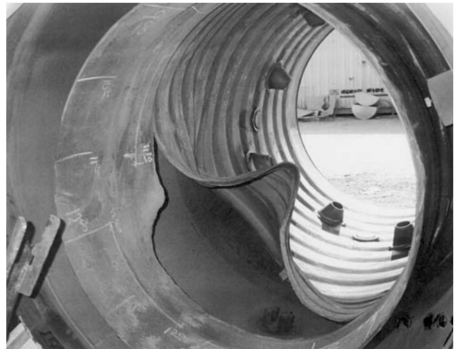
Figure 65. Major Rupture of Liner in a Silo Combustor.
