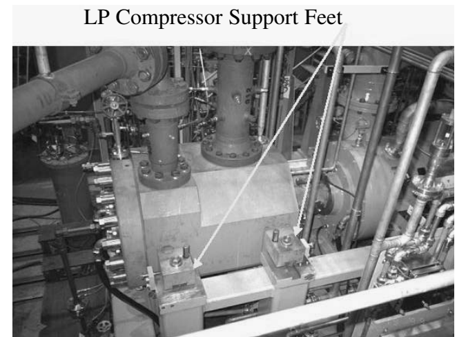
Figure 13. LP Compressor Support Feet.
