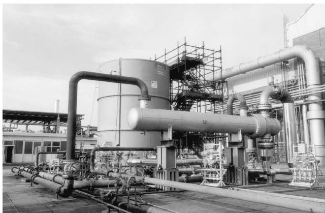
Figure 7. 850 KW (1139.87 HP) Subsea Compressor Module Facilities in Florence.
