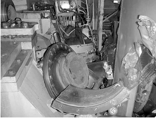
Figure 15. LP Turbine End to Generator.
