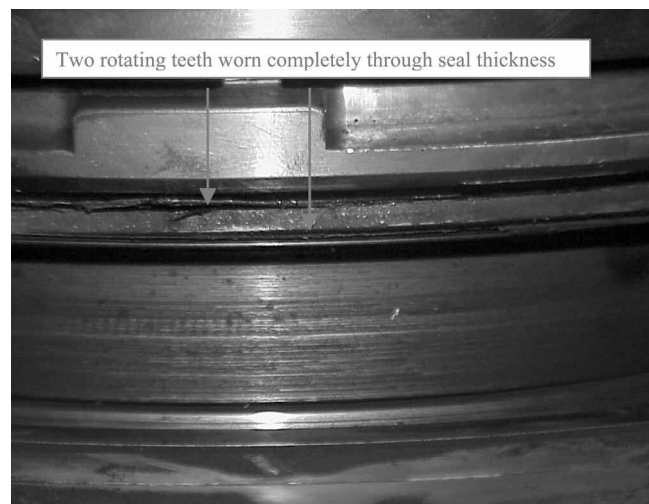
Figure 47. Damaged Buffer Gas Labyrinth Seal.
