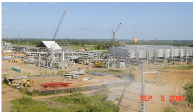
Figure 1. Construction of Boquerón Oil Field Facilities.
