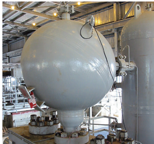
Figure 17. Fifth Stage Suction Sphere.
