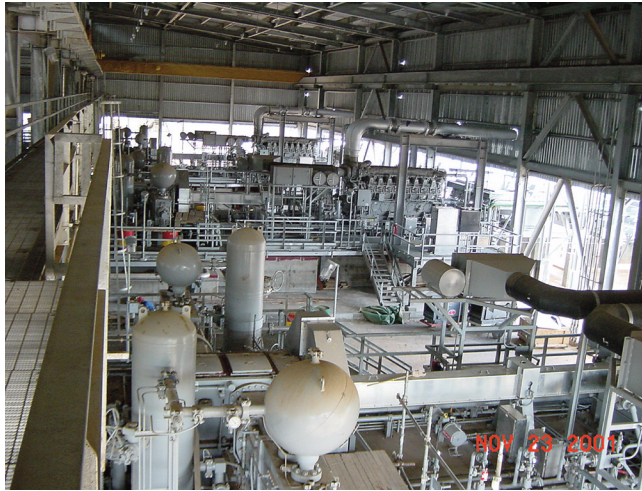
Figure 18. HP Injection Compressor—Phase 1 Installation.
