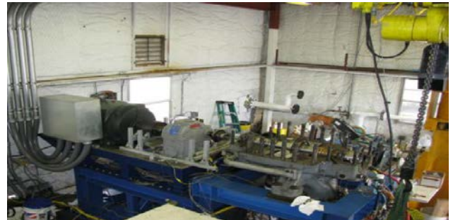
Figure 8. Compressor Drive Train
