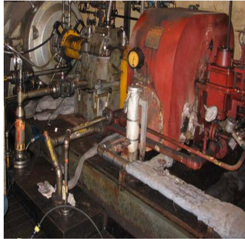
Installed 3/4" Adhesive anchor bolts at approx. 12" apart on the base plate
