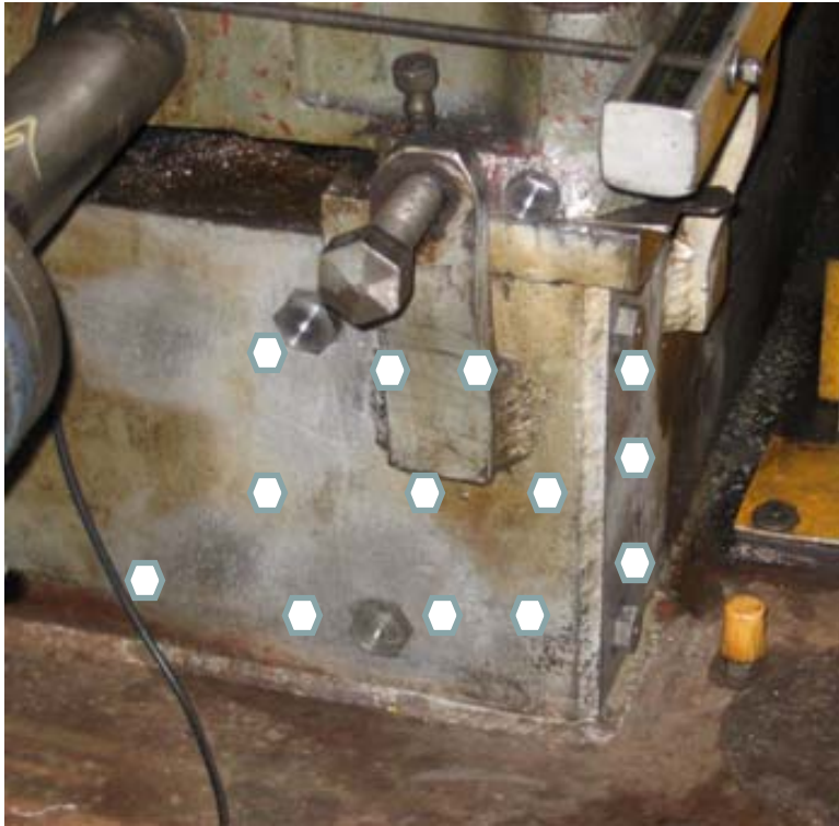
Installed 1/2" Adhesive anchor bolts at approx. 4" apart
