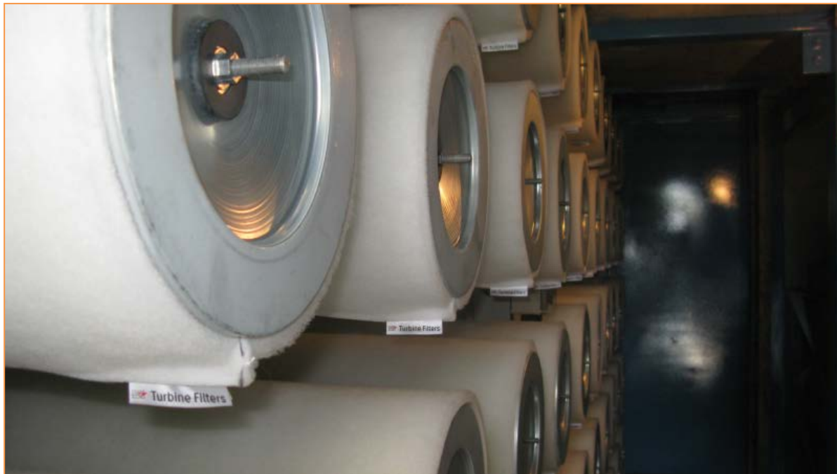
Cylindrical/conical hydrophobic HEPA filters with coalescers installed in refurbished inlet filter house.
