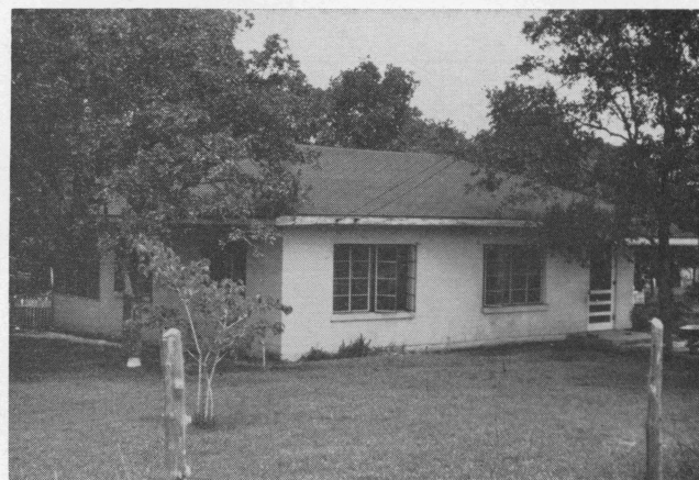
Figure 2. Photograph made when the family moved into the house.
