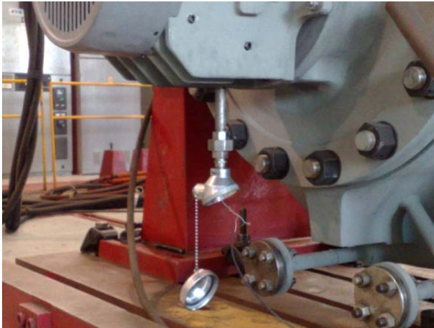
Figure 2. RTD for Bearing Oil Sump Temp. Measurement
