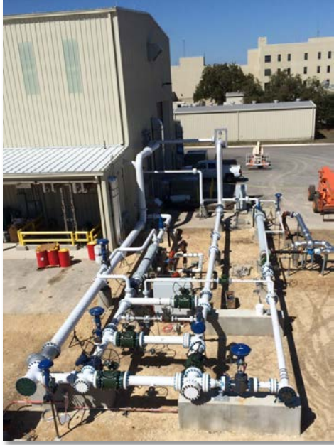
Figure 4. Pipe Loop Assembly Aerial View
