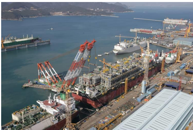
Figure 2. Agbami FPSO at the fabrication yard in Korea.
